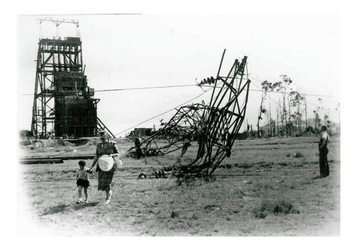
The tornado struck the Durban Deep Mine headgear and pylons and cables south of Roodepoort town early on, plunging the town into darkness. The electricity supply being cut off was actually a positive thing – not a single fire broke out. There were also no electrocutions reported because no electrical wires trailed across the streets.
